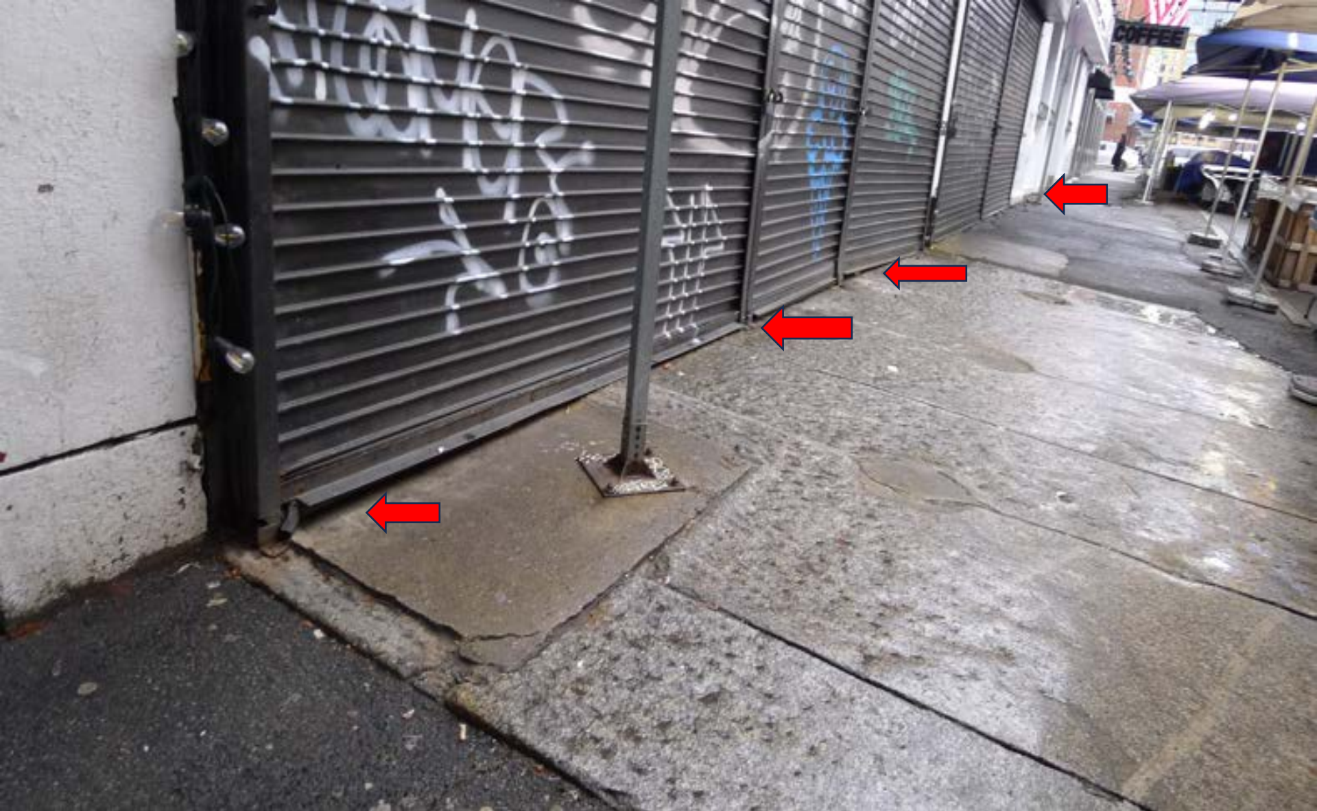
Figure 34. In addition to the rat proofing of the sidewalks, all doors all along the Haymarket neighborhood must be rodent-proofed, otherwise rats will move indoors and live in walls but forage outdoors during market days and nights. There are professional-level door seals that should be installed on each of these doors. (e.g., www. Xcluder.com ).
