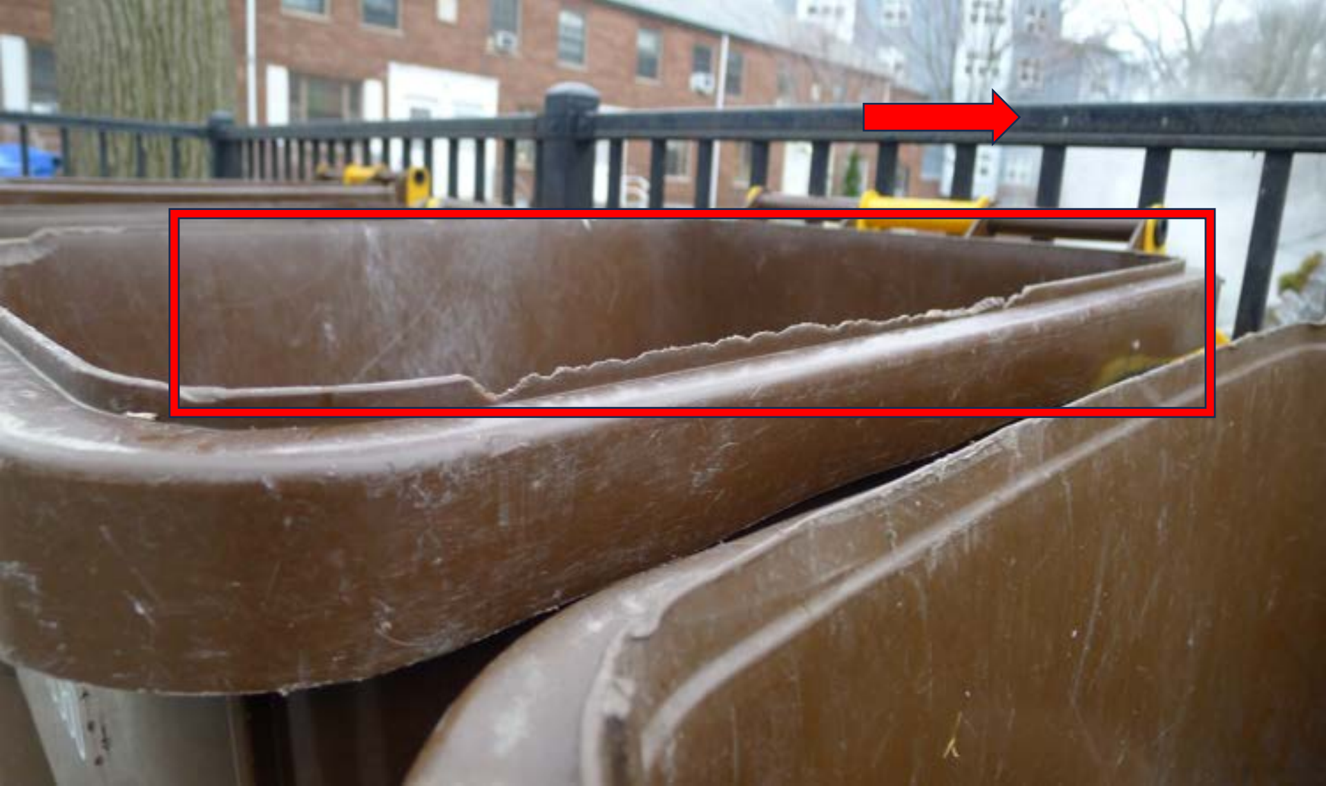
Figure 48. This BHA property's rats had no difficulty in climbing the gate rods and gaining access to the plastic garbage cans for food as seen by the evidence of the rats perching on top of the cans and gnawing apart the lid tabs. The gate and the cans themselves are covered in rat urine and rat body grease (called rub marks). Such is a concern from a public health perspective since human hands will surely have occasional contact with these same surfaces.
