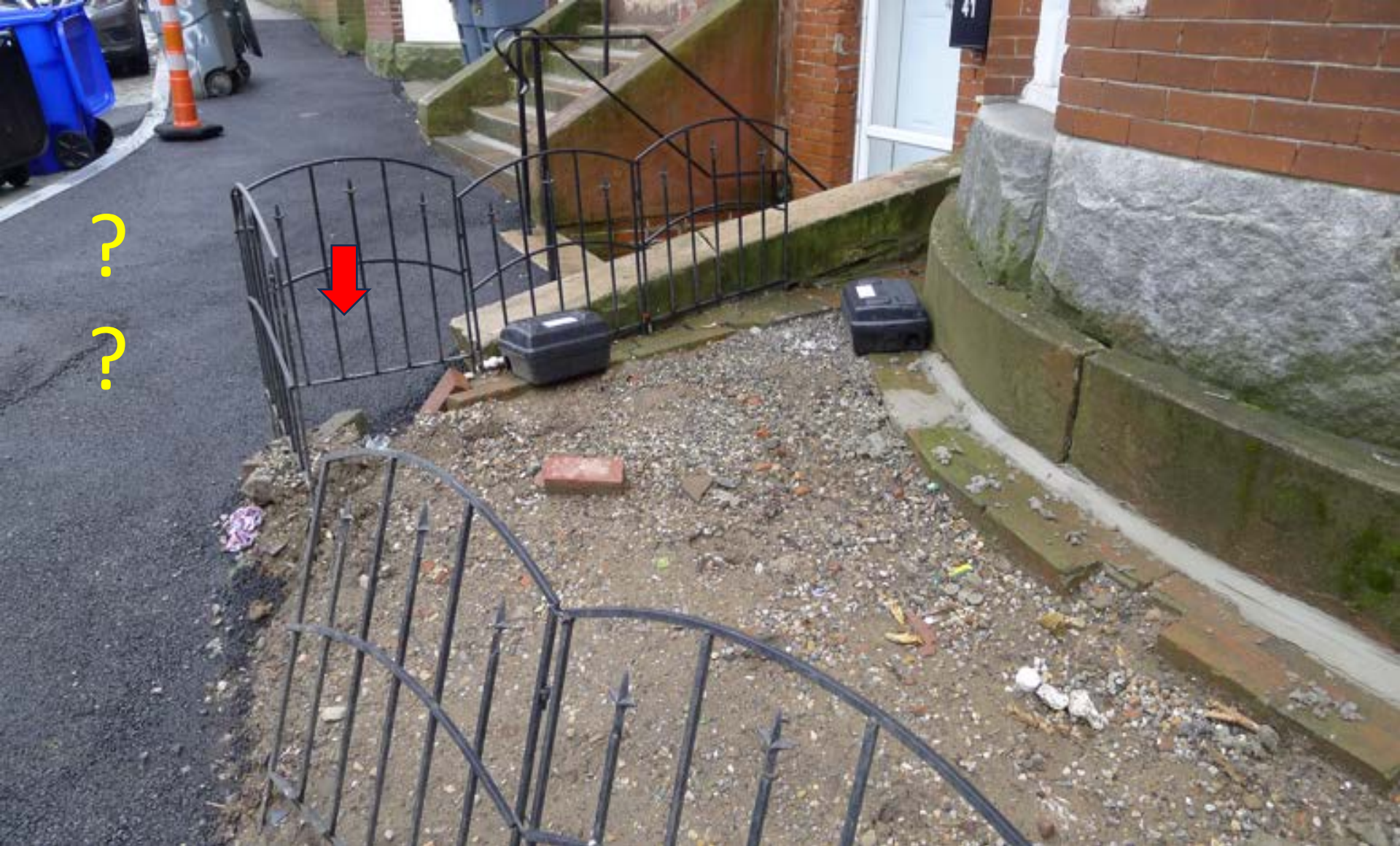
Figure 9. It was common to sight residential properties of Roxbury with severe rat infestations. Note this yard and the sidewalk (and the multiple bait stations trying to fight off the rats). The rats have burrows already constructed beneath the new asphalt (red arrow). How much of this entire new asphalt sidewalk is due to previous rat burrowing/destruction? (Also see Figures 78-79).
